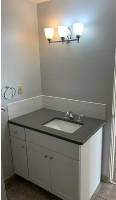
new sink and cabinet
